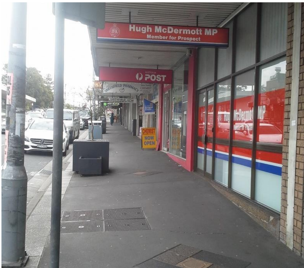
Figure 6.4: Smithfield shops looking west.
