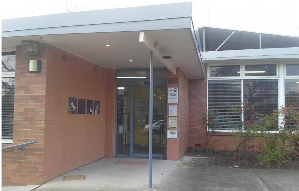
Figure 6.12: Smithfield Community Library, 57 Oxford Street Smithfield.
